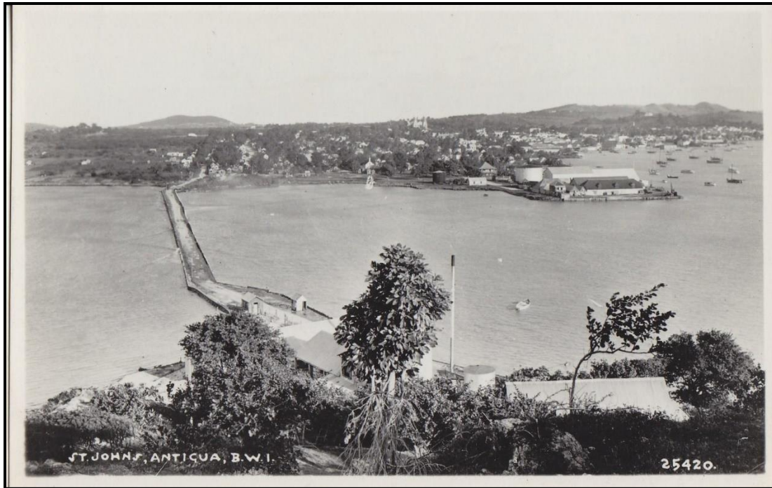
Rat Island causeway. Date unknown but note the gate houses.
